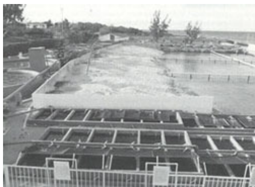
Figure 14.2 Part of the facilities of Cayman Turtle Farm, (1980's) showing screened hatchling tanks in the foreground, the Farm's breeding pond and adjacent beach with visible turtle tracks, and 9m diameter concrete stone block stock tanks on the left. The farm's hatchery is distinguishable in the background.
